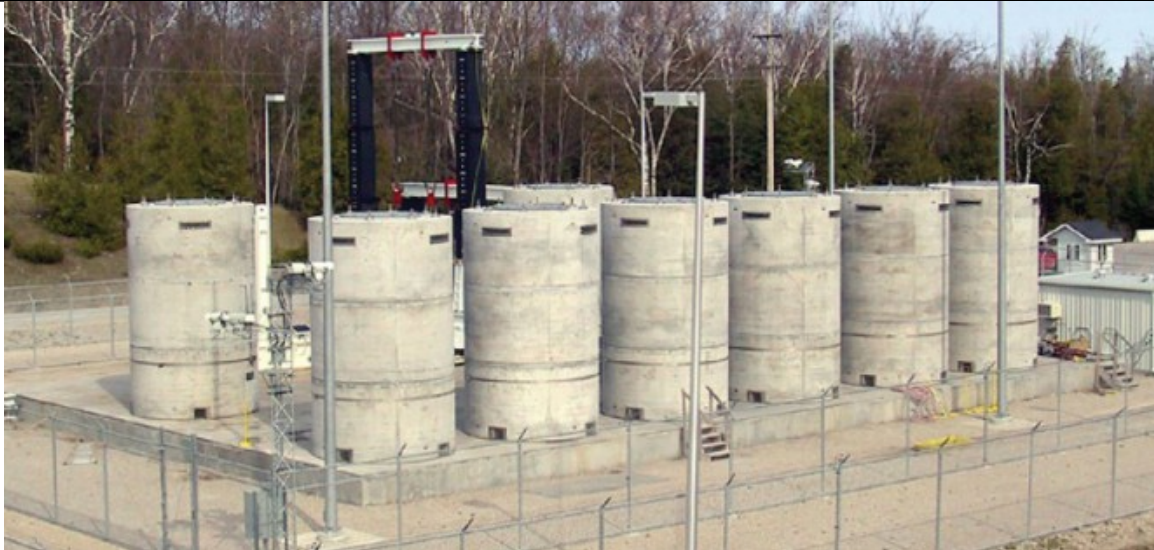
High Level Nuclear Dry Cask Storage at Big Rock Point, Traverse City, Michigan.
